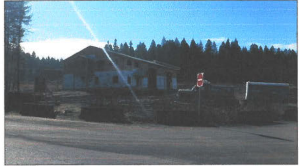
Neighbouring property to the north – currently under construction.
